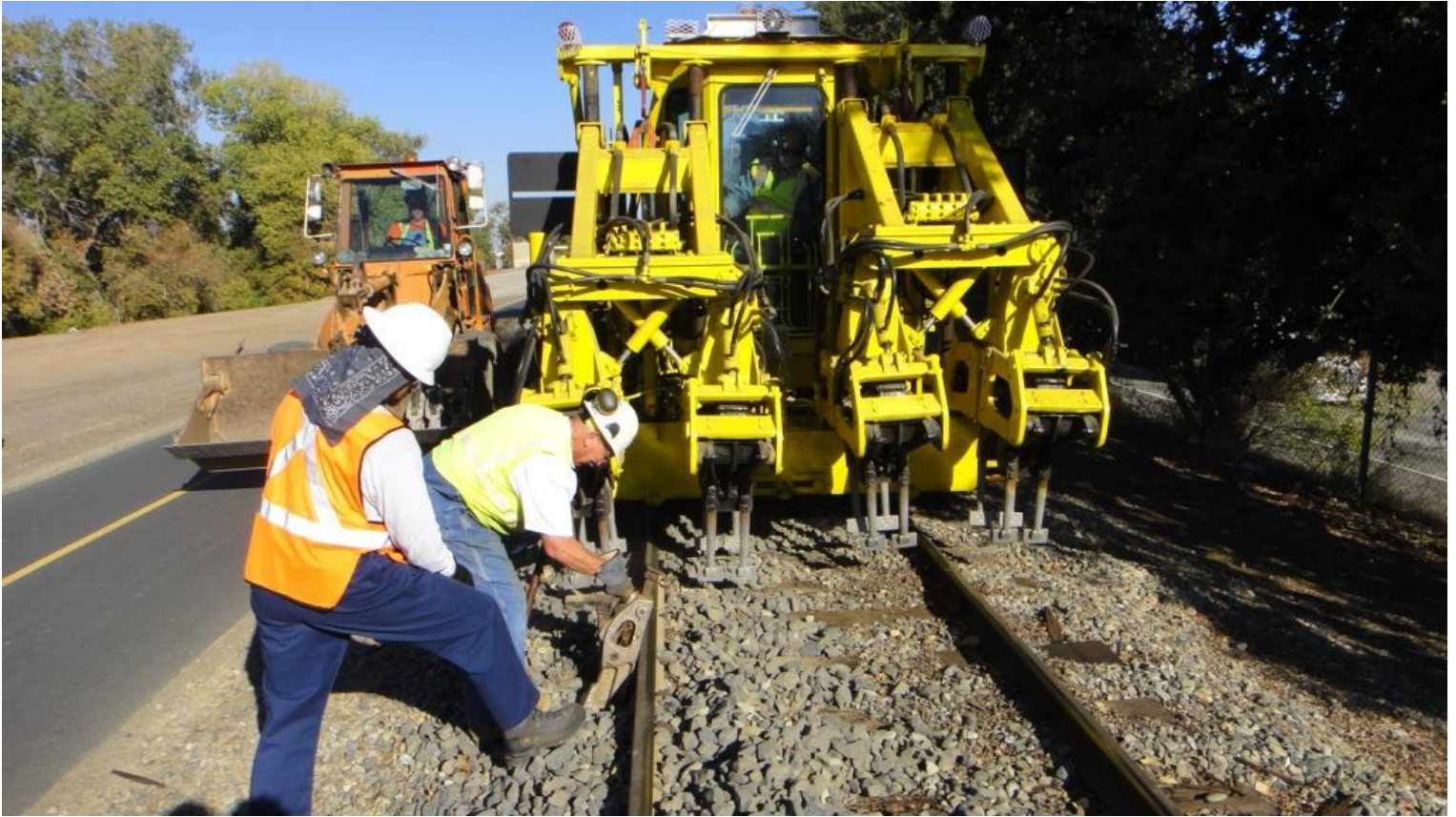
Clem and Jose pull the jack as Alan in the tamper tamps the west rail to level
