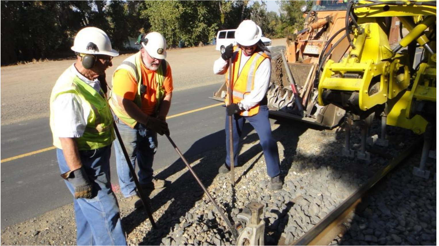
Frank nips-up a tie as Clem and Jose use lining bars to jam rock under it
