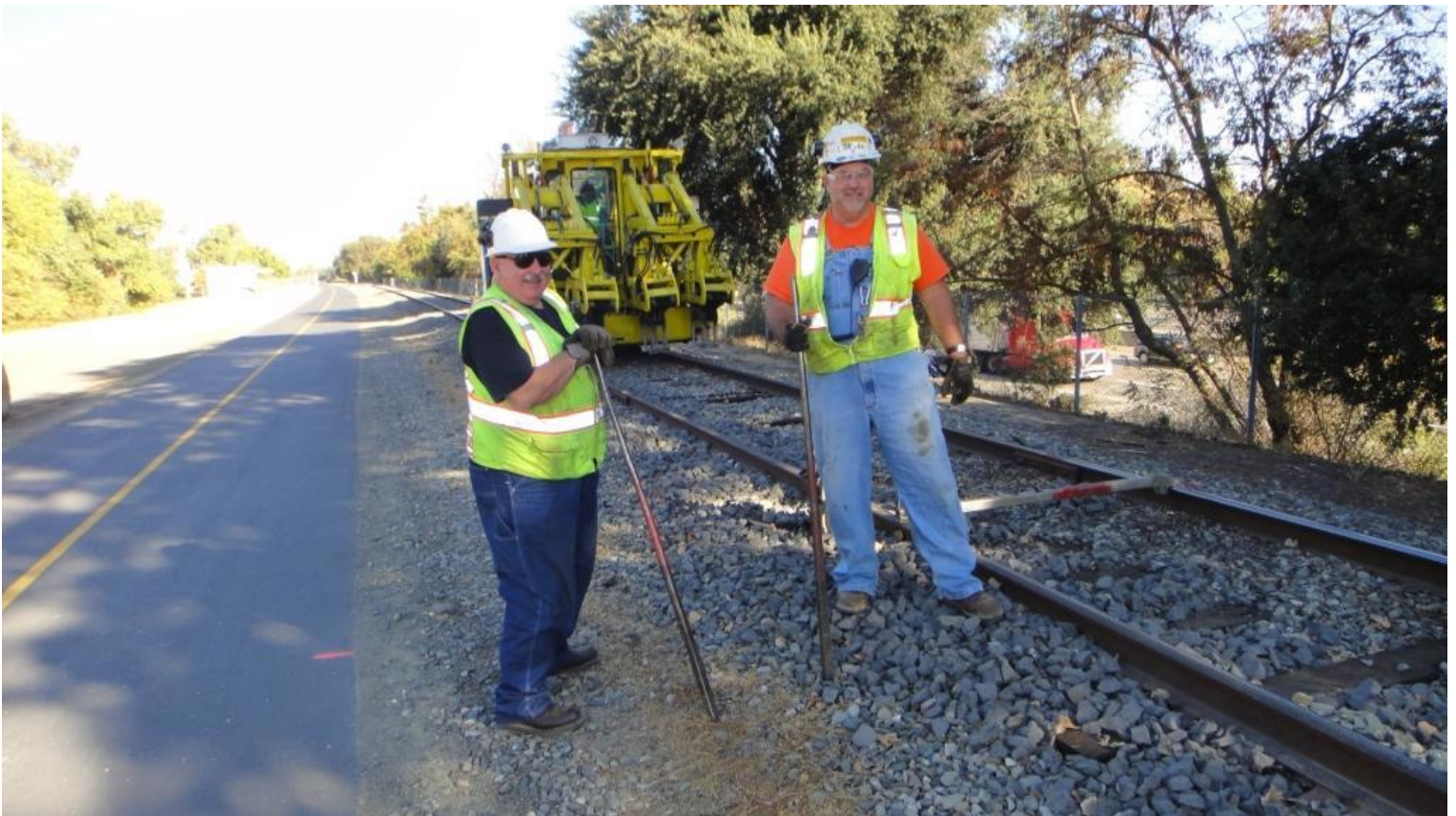
Harry and Mike F. with lining-bars in hand stand ready and willing to start jacking the west rail
