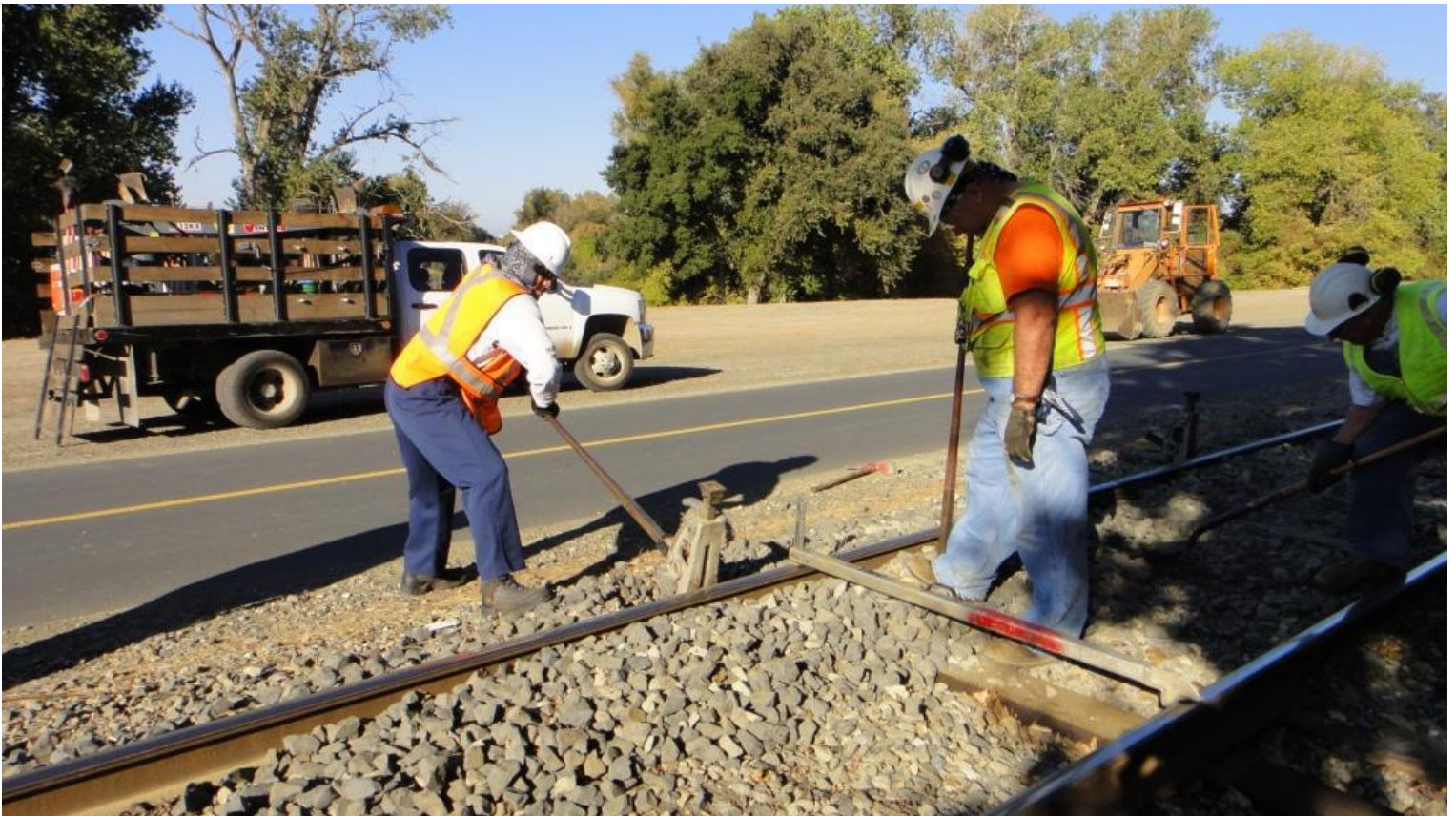
Jose jacks the track as Mike F. checks the level
