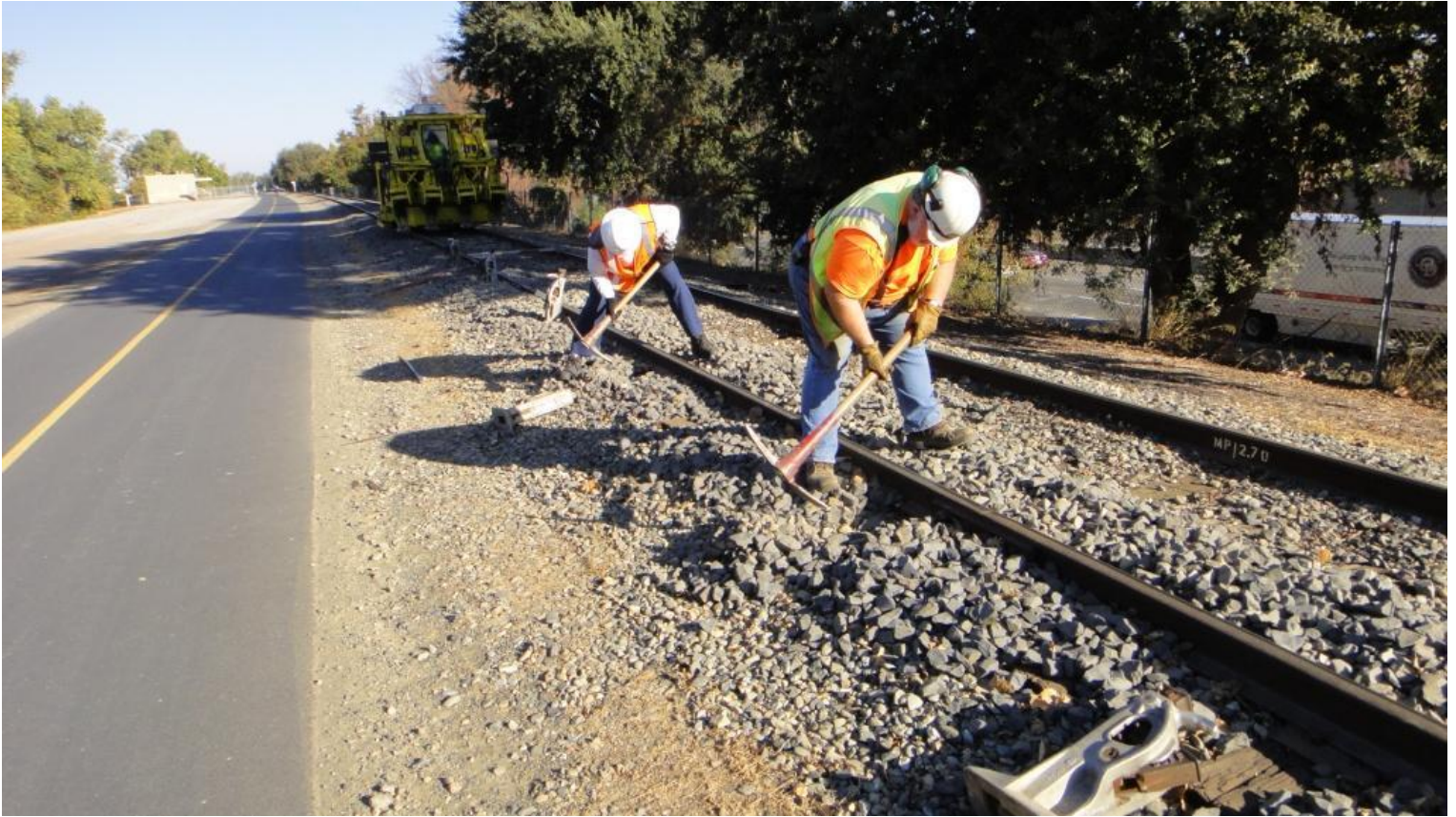
Jose and Frank dig-out spaces under the west rail in which track-jacks can be placed
