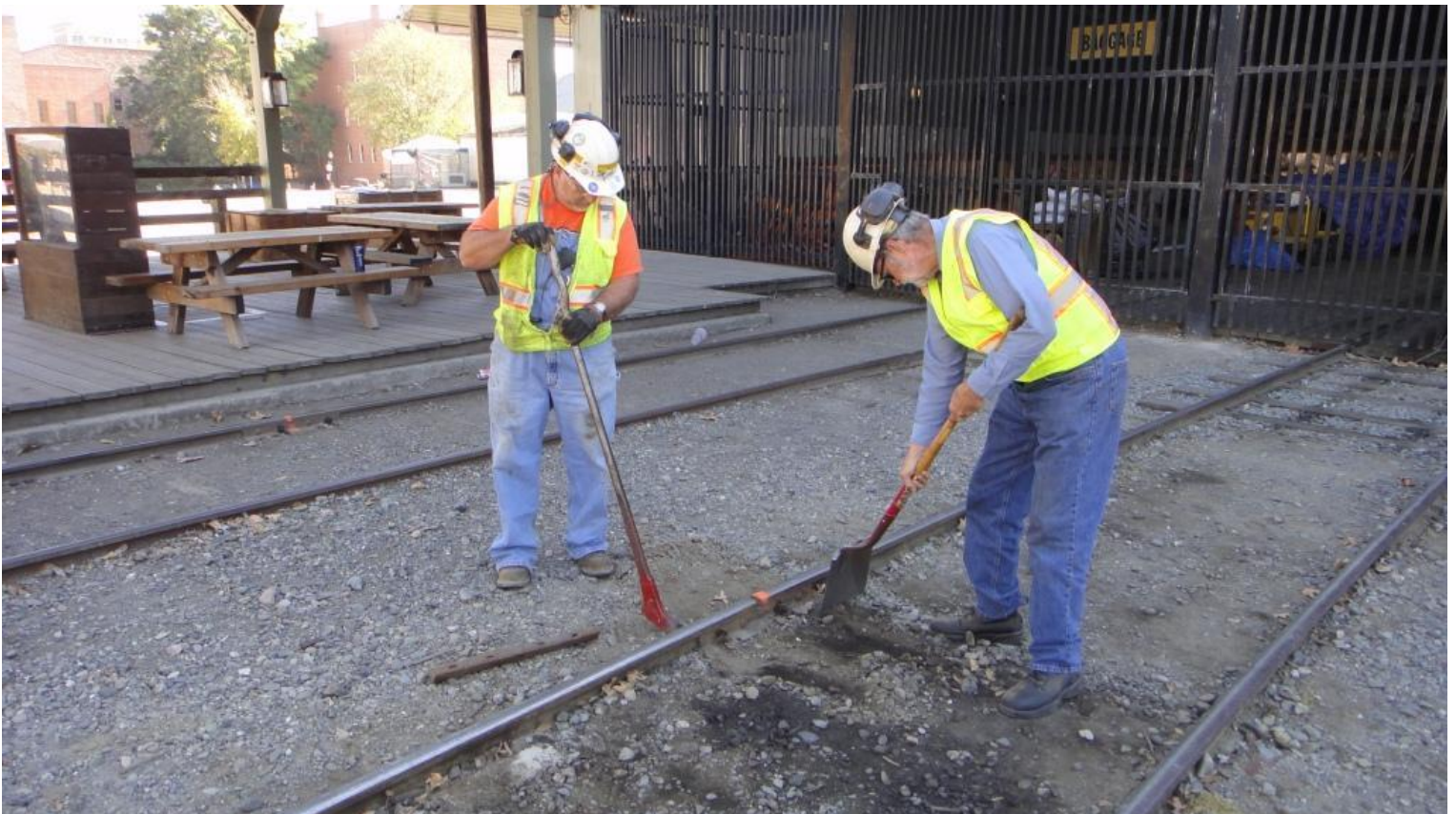
In the afternoon, Mike F. and Alan work on replacing a cracked joint-bar on Track 2
