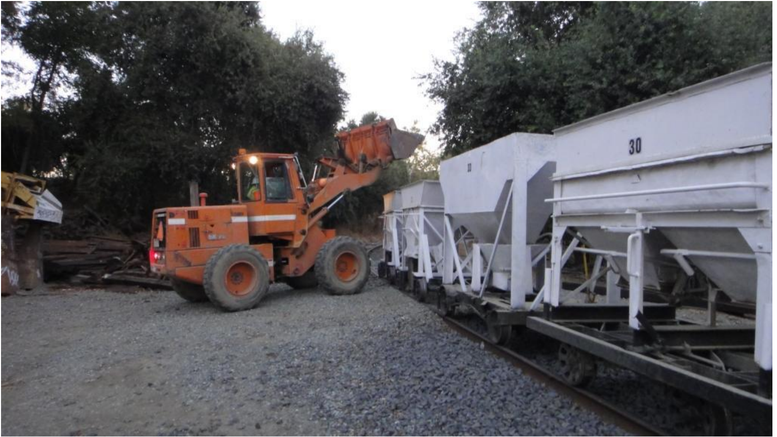
Mike H. in the front-end loader loads rock into the side-dump hoppers
