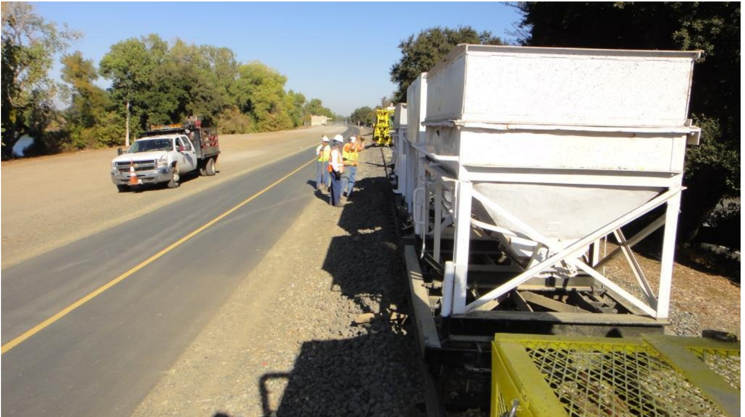
Frank, Clem, and Jose ballasting the track
